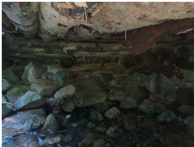
Left Bank Abutment when facing downstream
