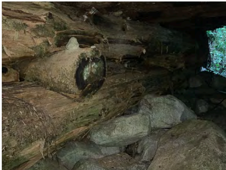
Right Bank Abutment when facing downstream
